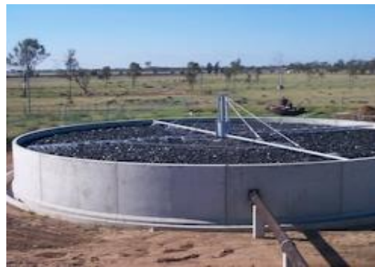
A schematic diagram of standard rate trickling filter
