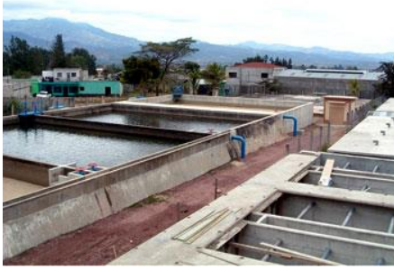
slow sand filter with water layer
