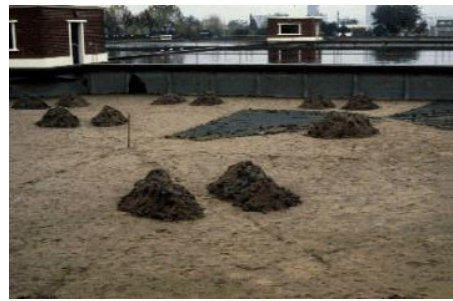
Removal of dirty skin layer
