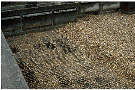
Under drainage system of slow sand filter
