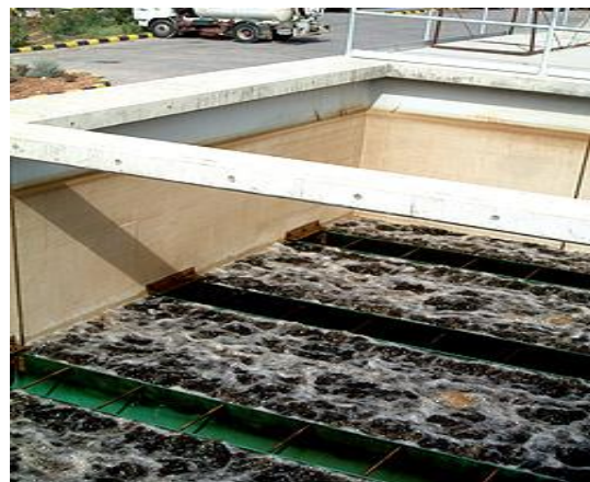
Rapid Sand Filter Back-wash and Air-wash type
