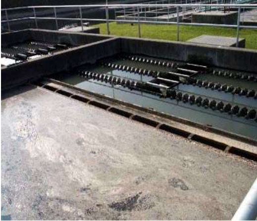
Effluent weir of rectangular sedimentation tank
