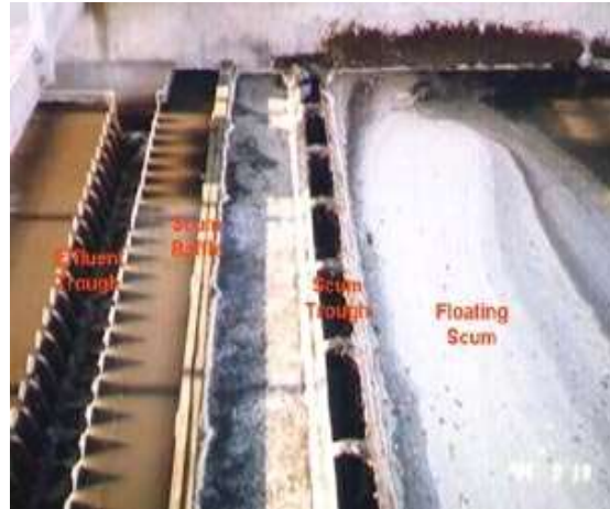
Effluent weir of rectangular sedimentation tank
